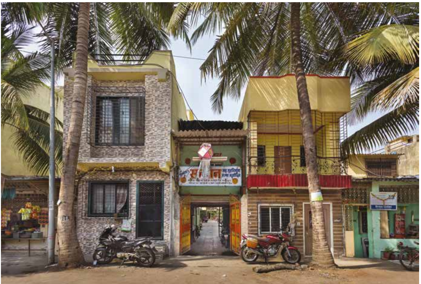
The formal entrance to one of the many housing courtyard clusters that define the Charkop Sites and Services Scheme, Mumbai. © Kunal Bhatia (Studio Kunal Bhatia) Sameep Padora & Associates
