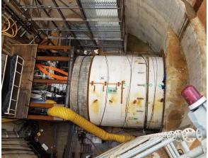
AlexRenew: Shaft excavation, TBM assembly and launch
