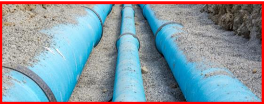
Utility Work: May 2021 – Jun 2021
