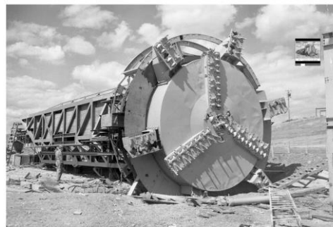
THE "MOLE" SHOWING ITS 26 FOOT CUTTING FACE, USED IN DIGGING UP TUNNELS AT SITE OF Oahe DAM NEAR PIERRE, S.D., THE DIGGER IS OWNED BY MITTRY CONSTRUCTORS OF LOS ANGELES AND IS 6-1/2 FEET HIGH, 105-4-10-21. 1353 1310.36 8-10-55
