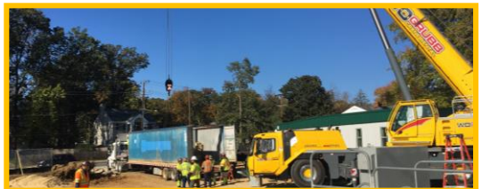
Crane On Site: April 12 - 16
