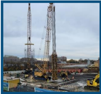
Support of Excavation
