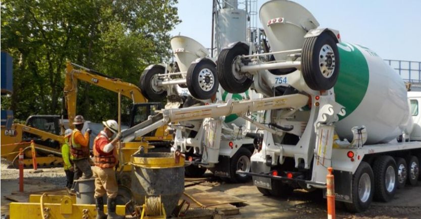
2,700+ cubic yards (~340 trucks) Concrete placed to-date
