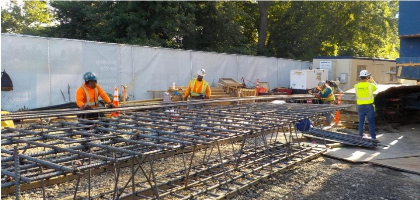
93,000+ pounds (46+ tons) Rebar installed to-date
