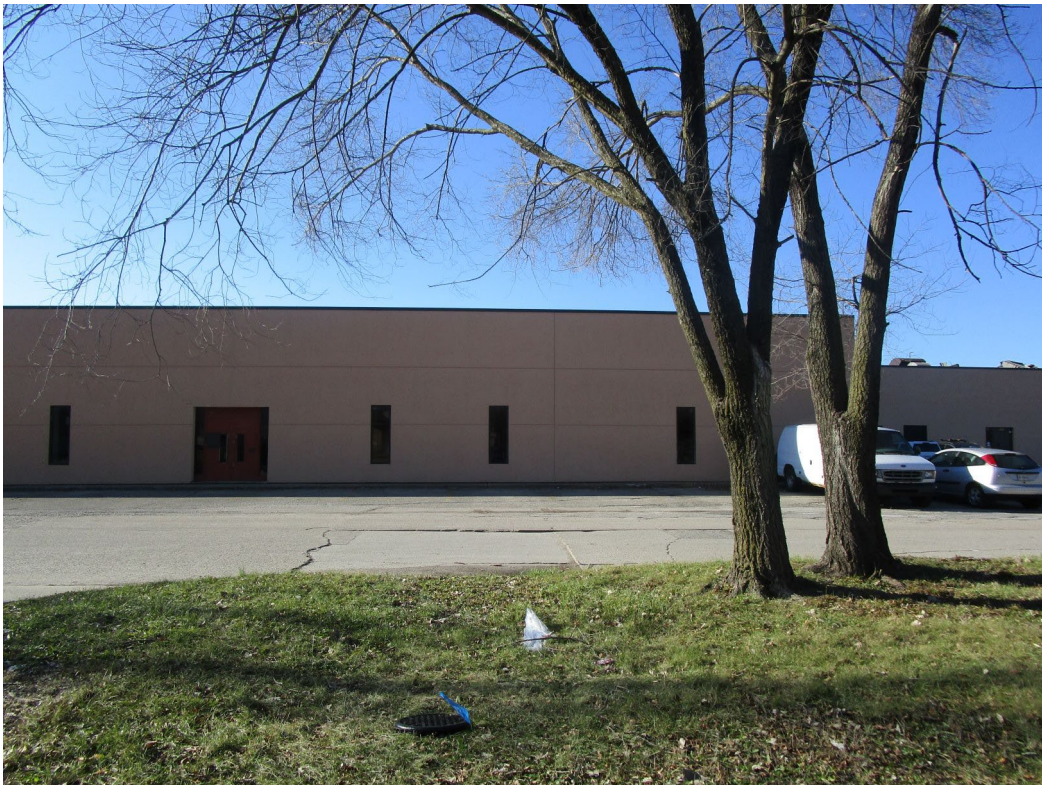
View from site looking west across South Kenyon Street
