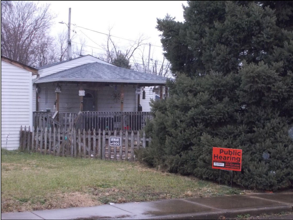
Looking northeast at the subject site from Beecher Street.
