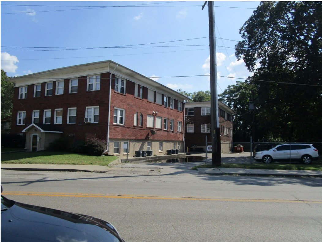
View from site looking south across Fairfield Avenue
