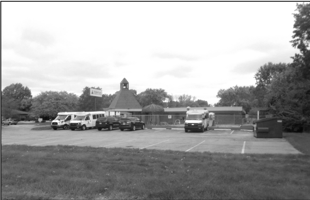
Looking north from Rockville Road at the neighbor to the west of the subject site.
