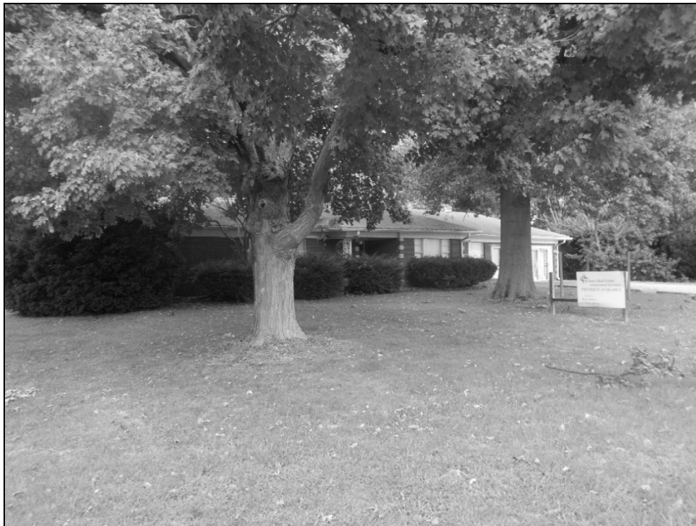
Subject site, 8850 Rockville Road.
