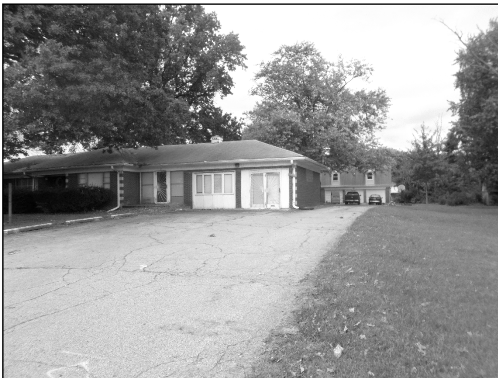
Subject site, 8850 Rockville Road.
