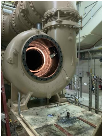
108 to 116: Upgraded pumps
