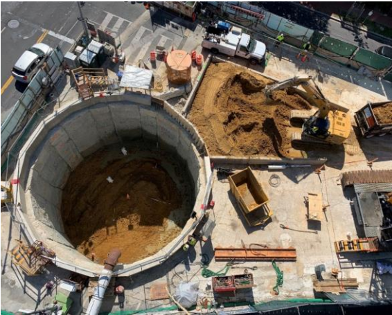
AlexRenew: Shaft excavation, TBM assembly and launch ! Noise variance for these phases approved
