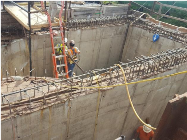
Hooffs Run Interceptor: Diversion chamber and open-cut sewer construction
