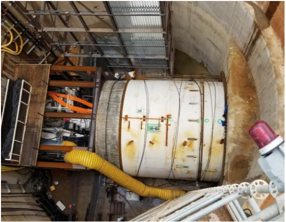
AlexRenew: Shaft excavation, TBM assembly and launch ! Noise variance for these phases approved
