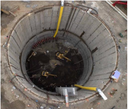
Royal Street: Shaft slurry wall construction and excavation ! Noise variance for these phases approved
