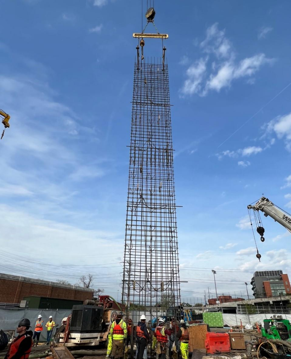
Rebar lifts may temporarily impact traffic in cul-de-sac and bike path
