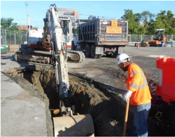
Hooffs Run Interceptor: Diversion chamber and open-cut sewer construction
