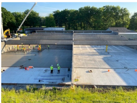
Ranges 1 and 2 – Cement installation
