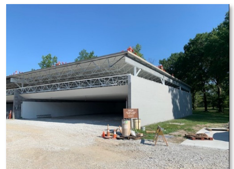
East Tac Bay – Roof installation, painting complete
