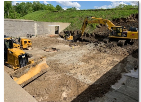
Range 1 – Berm reduction and foundation excavation
