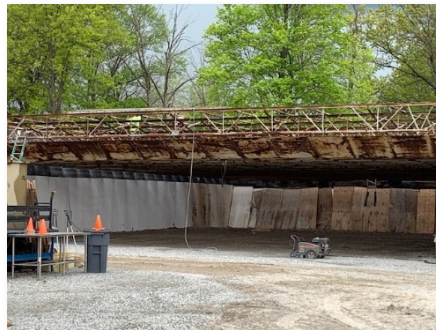
East Tac Bay – Day one, steel remediation
