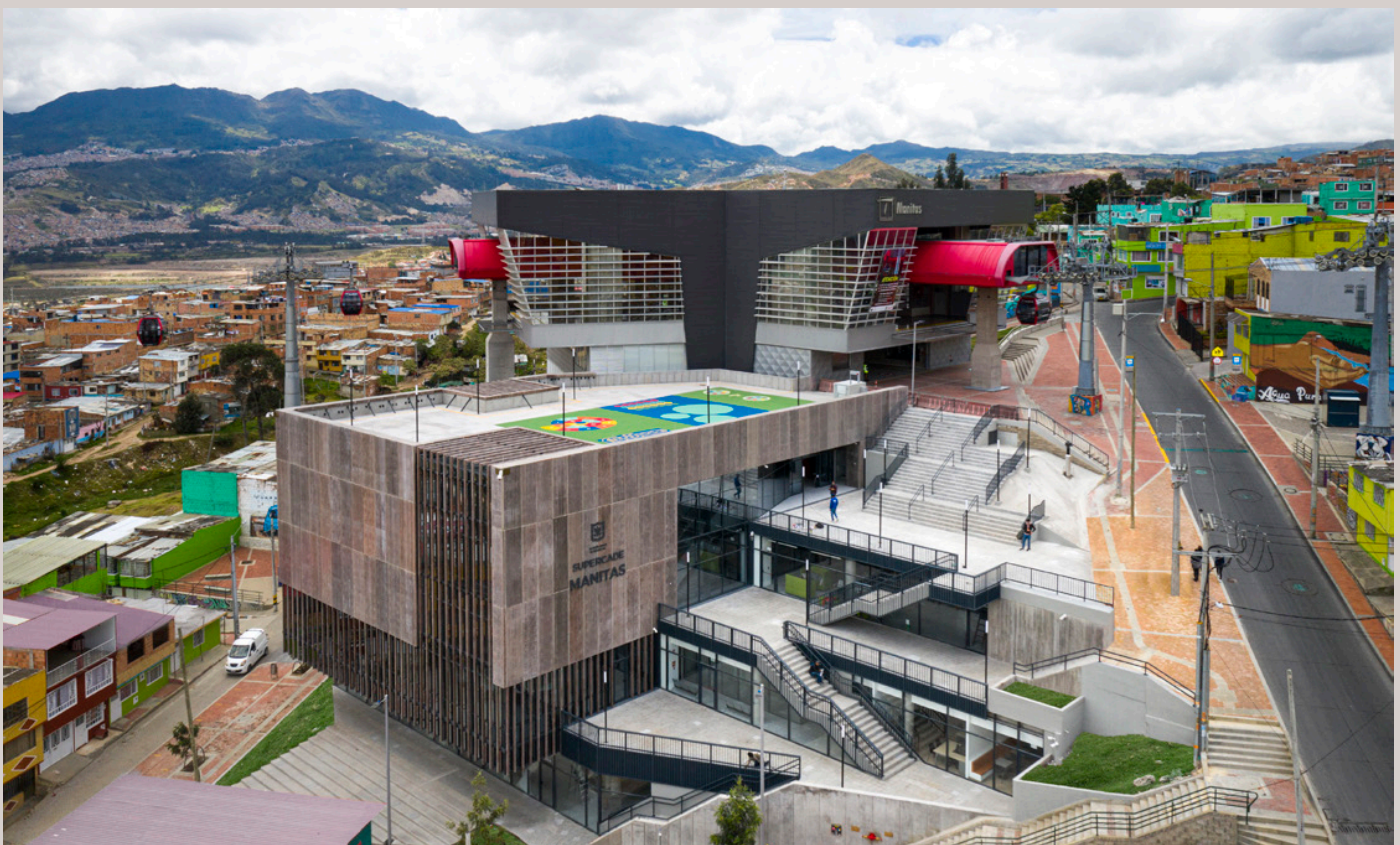
The Ciudad Bolívar Care Block is housed within the SuperCADE building © Ilanofotografía
