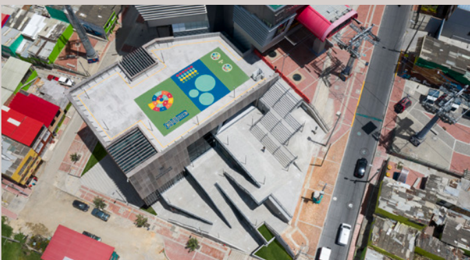
The roof of the SuperCADE acts as a public space for caregivers and the surrounding community © Ilanofotografia
