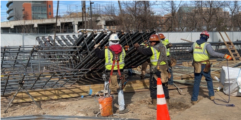
650,000+ pounds (325 tons) Rebar installed to-date
