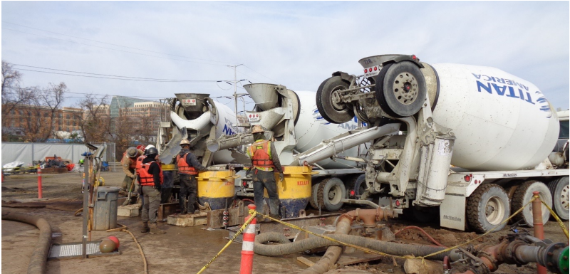
15,000+ cubic yards (~2,000 trucks) Concrete placed to-date
