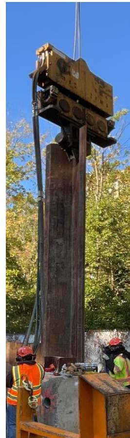
Vibrate piles initially
