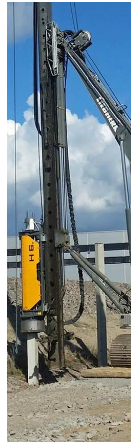
Evaluate use of hydraulic vs diesel hammer
