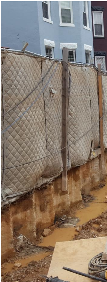
Sound blankets along fence to dampen noise
