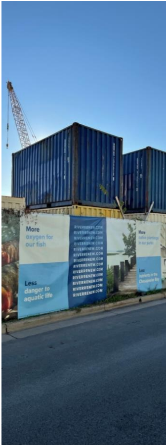
✓ Stacked conex boxes to deflect noise away from the community.
