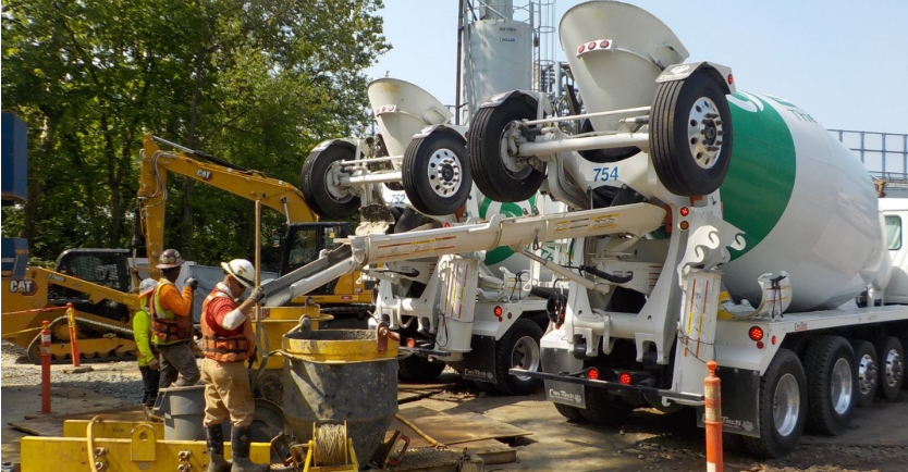
3,500+ cubic yards (~438 trucks) Concrete placed to-date
