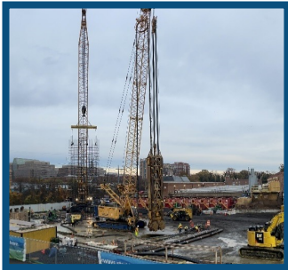
Support of Excavation
