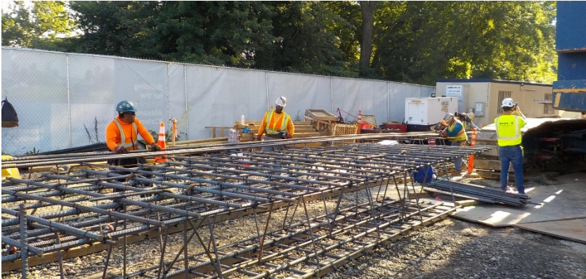
113,000+ pounds (57+ tons) Rebar installed to-date
