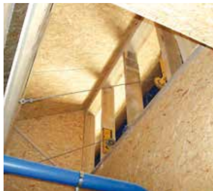
16 Recirculating air flap
