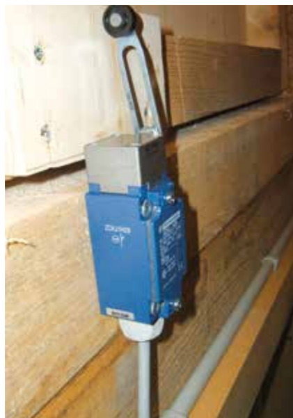
17 Air flap limit switch
