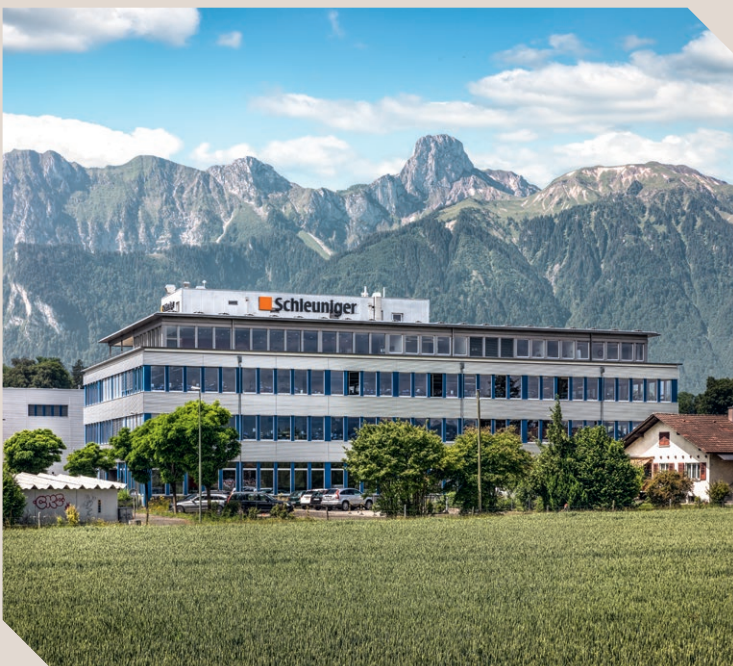
Schleuniger Group headquarters in Thun, Switzerland.
