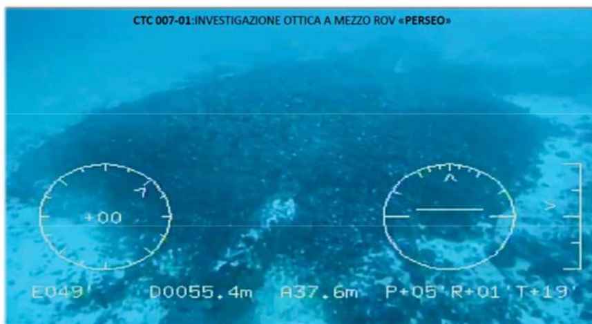
Figure 12: Image acquired with ROV of the Italian Navy, representing the concrete pour deposited to restore the accidental damage that occurred on the Transmed on December 19, 2008. Navy Archives.
