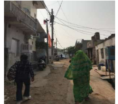
Fig 155 Main road of basti is not maintained proper.
