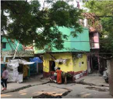
Fig 176 Open voids in between streets and houses
