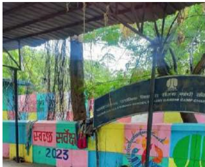
Fig 26 Existing situation of the school not in working condition with tangled wires , making it unsafe for children.
