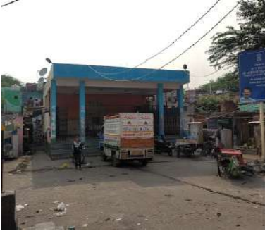
Fig 173 Community Centre in the basti have generous amount of space for functions and street vendors
