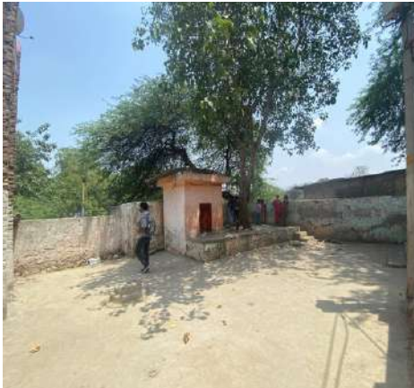
Fig 151 The existing Shiv Mandir has a lot of potential to be developed as a multiutility space for women and kids as a recreation area.
