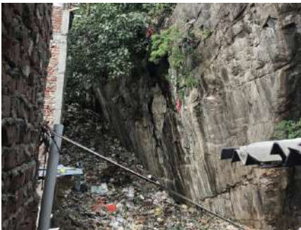
Fig 60 Solid waste is also dumped at open spaces in Basti.
