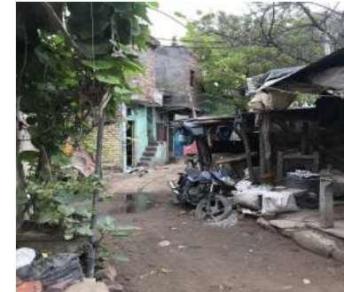
Fig 39 Pathway not proper constructed of Basti .
