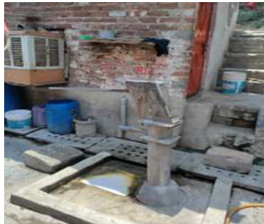
Fig 138 Hand pump boring is the major source of water in the basti
