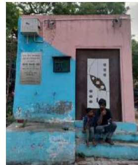
Fig 28 The water filtration R.O system currently not In use.
