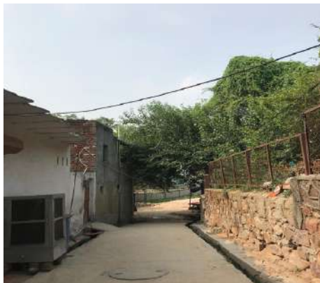
Fig 159 Sewage line is also present in basti.
