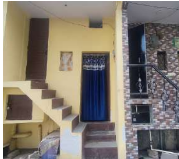
Fig 100 Space for Bore well motor connection for water.
