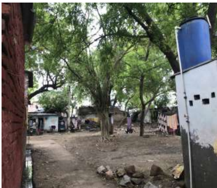
Fig 52 Existing situation of the open space in basti is not proper maintained and nali is not covered.
