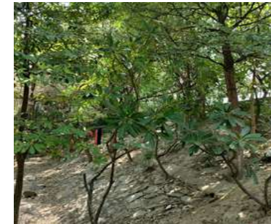
Fig 139 Road embankment covered with greens
