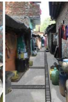
Fig 33 Reworking on the R.O.W as well as providing drain covers
