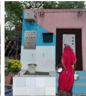
Fig 29 Reworking of the water filtration R.O system to bring it in use for free Potable water.
