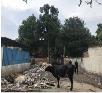
Fig 35 One more entry is also from railway officers colony side which is only pedestrian friendly which is mostly occupied by garbage and animals and the door width is very less.
