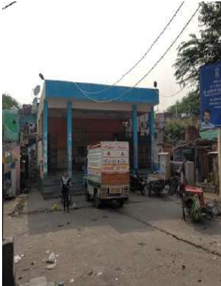
Fig 187 The existing Community centre has no metered electrical connection which makes it unsuitable for use.
