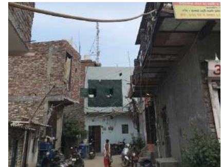
Fig 62 Entrance of the Basti with no proper water drainage and electrical poles.
