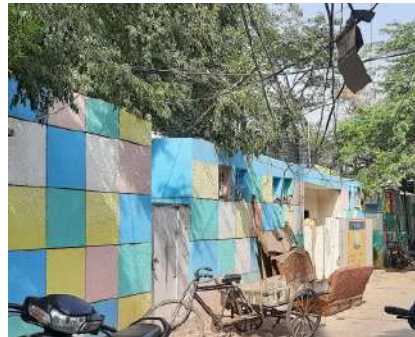
Fig 23 Public Toilet for both men and women
