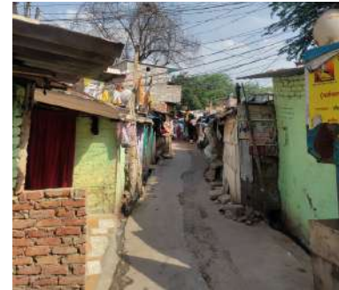
Fig 14 Lack of proper drainage and pedestrian friendly streets.
