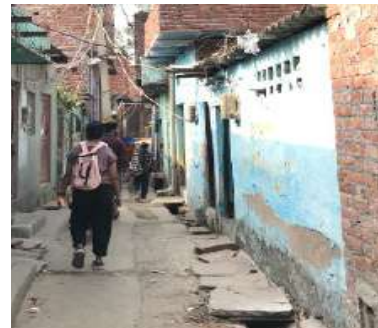
Fig 180 Drainage channels are present along every street in basti and almost every drain is covered.
