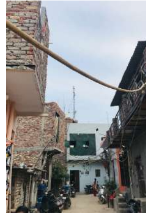
Fig 76 The existing entrance to the basti does not have proper drainage and also lacks electrical supply through poles as cluster of wires can be seen.
