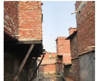
Fig 181 View of settlements built in the edge of nullah.
