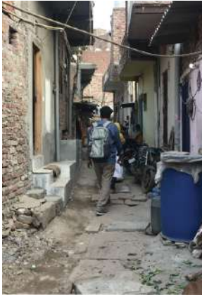
Fig 74 The existing streets of the Basti do not have proper drainage system.
