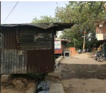
Fig 84 The drainage channels are present along every street.
