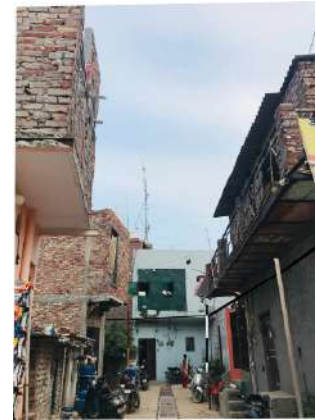
Fig 77 The proposed entrance to the basti includes proper drainage by working on R.O.W also provision for electric poles with safe wiring system.
