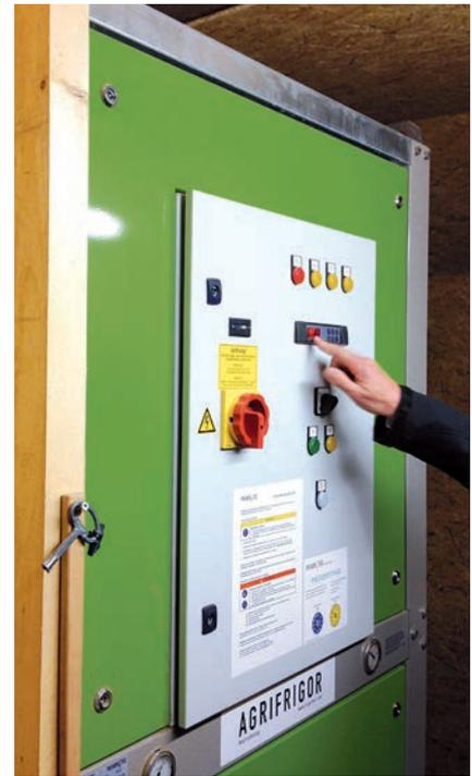
14 Heat pump (dehumidifier), FrigorTec factory image
