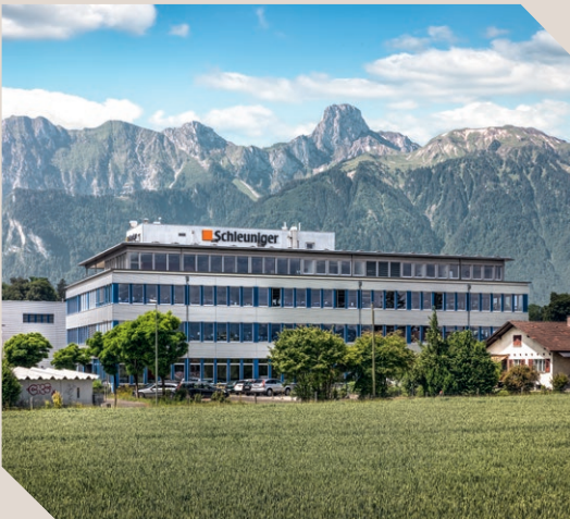
Schleuniger Group headquarters in Thun, Switzerland.
