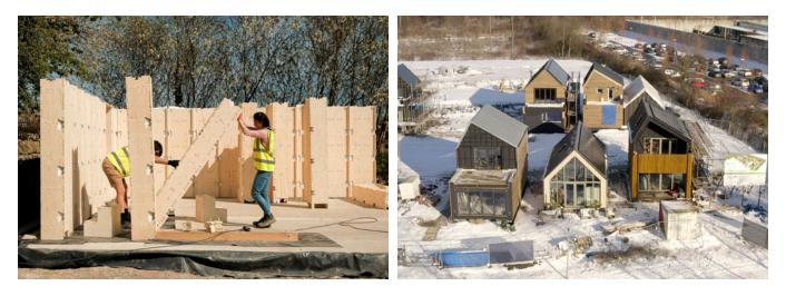
Wikihouse wall blocks being erected, Peaks Barn construction, UK (image credit: © Jack Watts (left)). Aerial view of the De Stripmaker neighbourhood, Netherlands, with nine WikiHouses under construction (image credit: © WikiHouse NL (right)). every policy and programme, from property taxation to housing income support and from land use to healthcare, is geared towards housing for the common good (Mazzucato and Farha, 2023).
