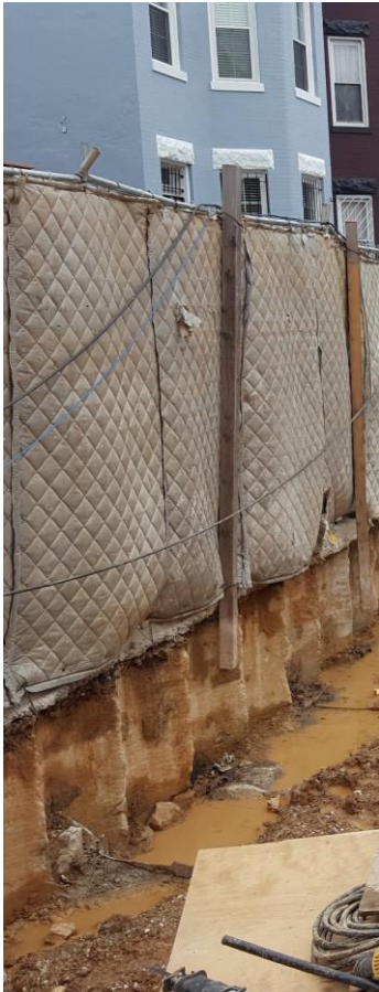
Sound blankets along fence to dampen noise
