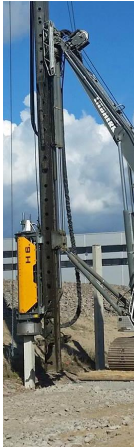
Evaluate use of hydraulic vs diesel hammer
