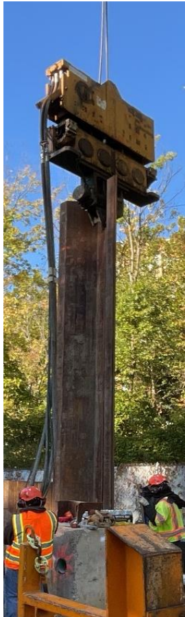
Vibrate piles initially
