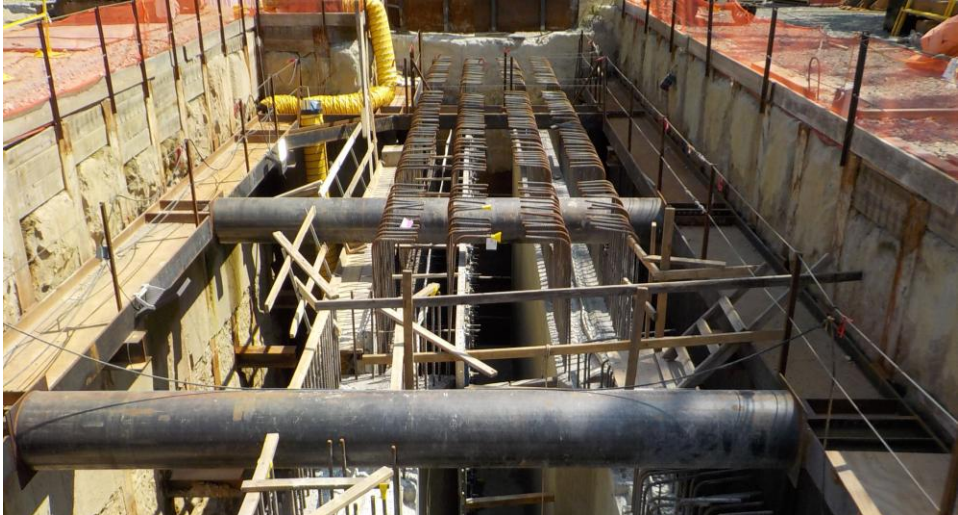
Support of Excavation for Diversion Facility
